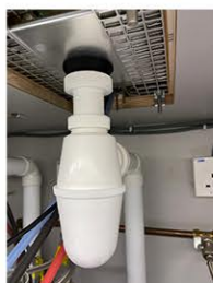
Optional - drainage point with bottle trap (connection to be completed by your contractor)
